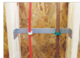
RSWB used in floor joists
