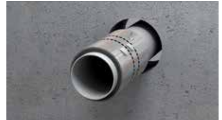
3. Bend and lock the tabs.
