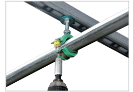
Tighten clamp to complete installation
