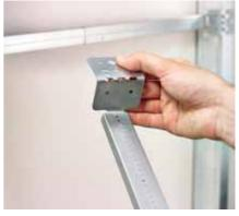
3. Bend the fixing plates along the markers, if required, for multiple depth settings.
