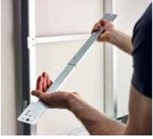
2. Slide the brackets together to the required length.
